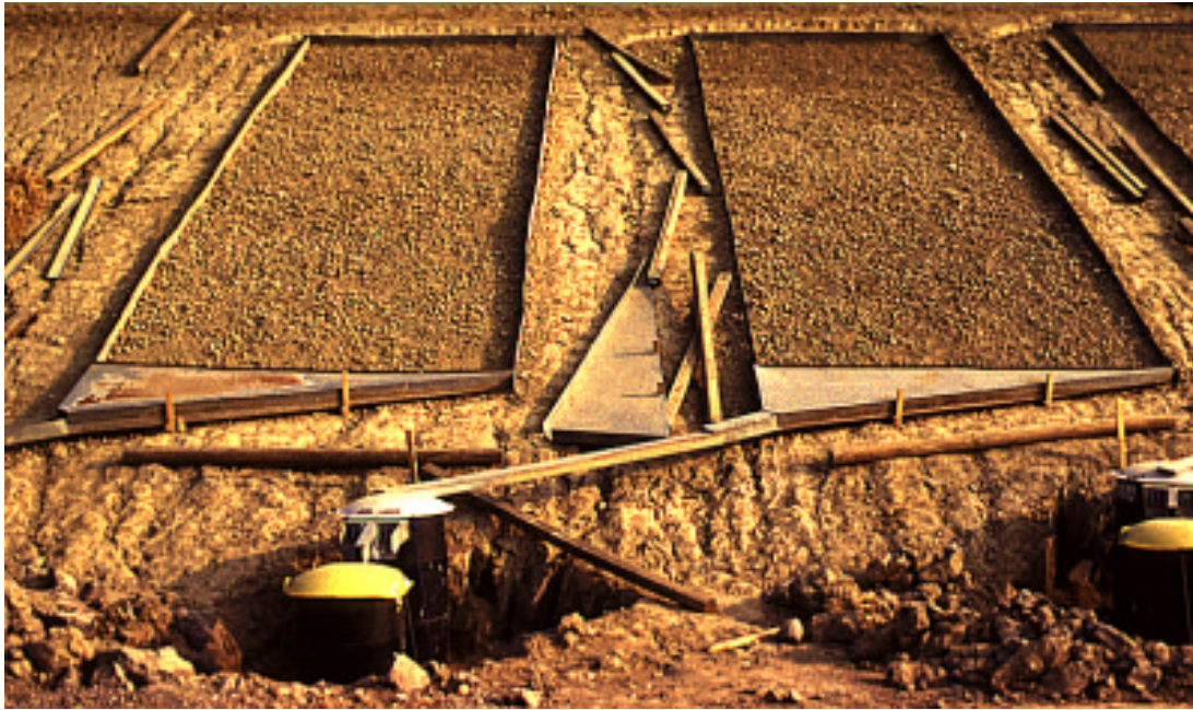
Figure 1. Typical plot setup for the natural rainfall studies, showing the two-barrel runoff collection system.
